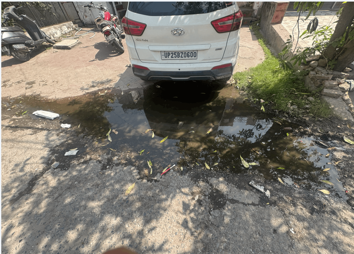
Fig 2 — Stagnant drainage water pooling beneath and around parked vehicles in residential areas. Dark water colour indicates contamination — probable sewage mixing with surface drainage.
